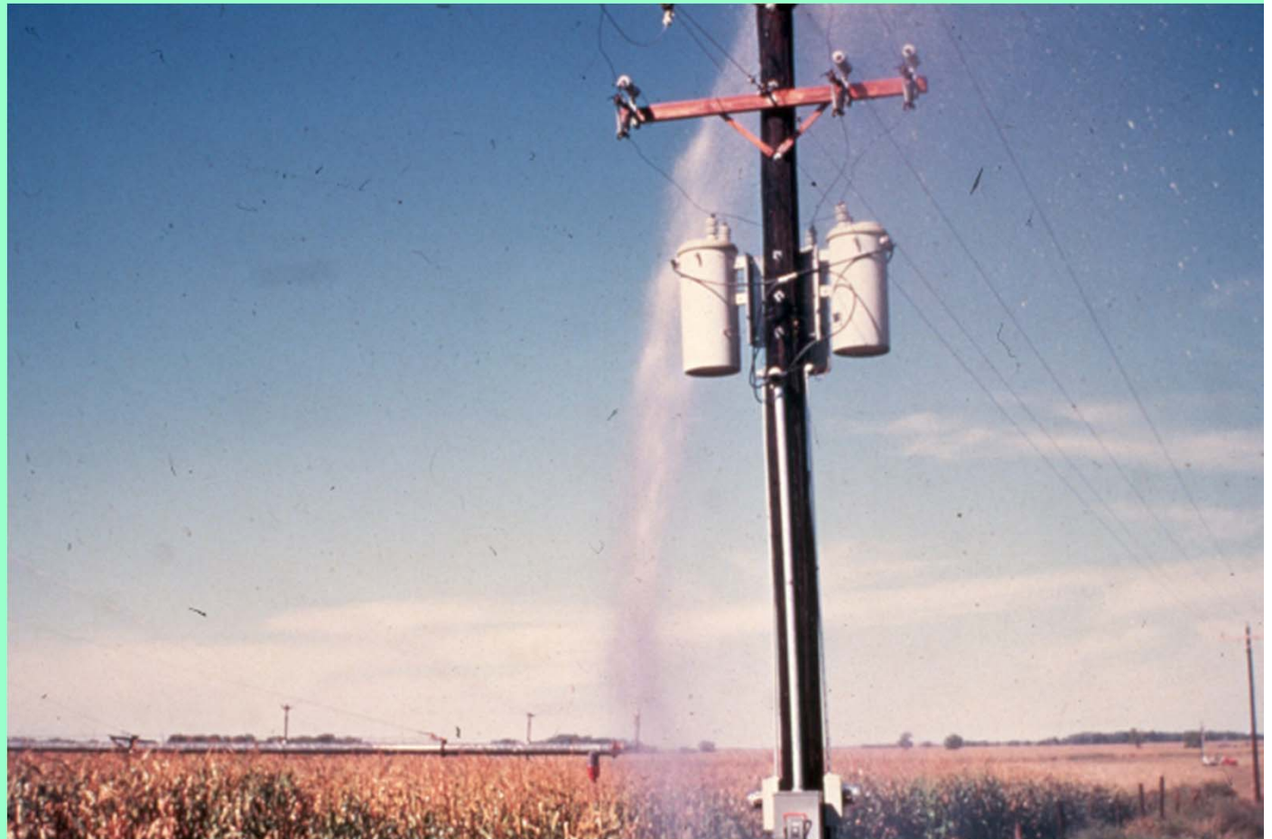
End gun spraying power lines & transformers
